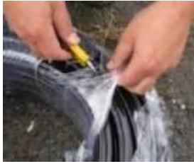
Open plastic wrapped rolls carefully! Blades or knives can easily puncture the airline. If the airline becomes cut, cut the tubing on each side of the damage and use clamps and connectors to splice the ends together.
